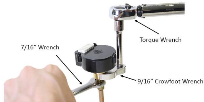
Figure 2-6 USHX Installation with Torque Wrench (70 in-lb)
